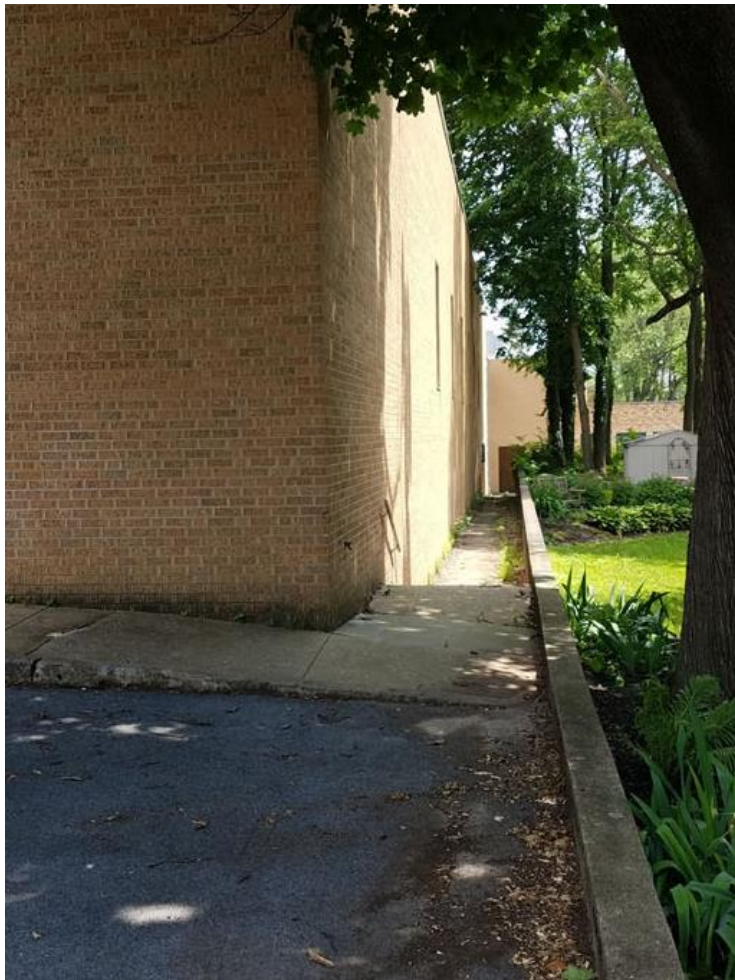
Wall along residential property boundary
