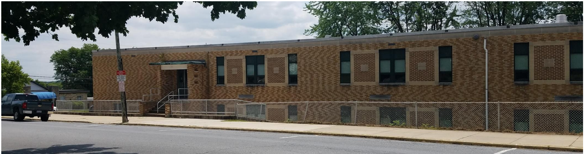
Walnut St. façade – 1965 two-story structure, cut into hillside, approx. 20' above Market St.
