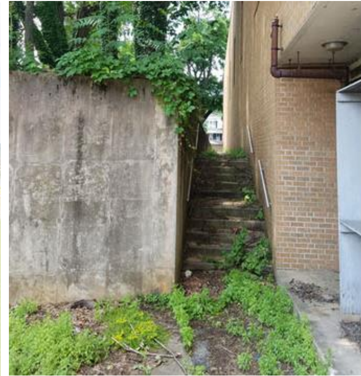
Stairs / retaining walls
