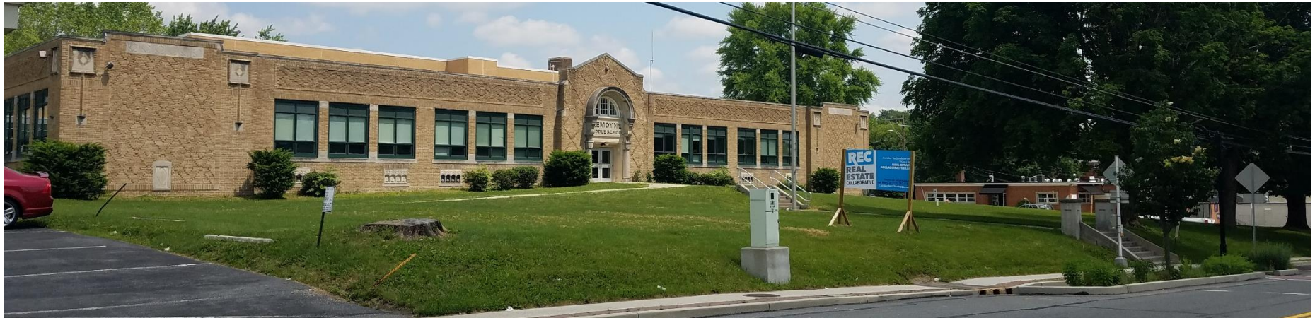
Market Street façade –1925 building, architectural features, front lawn, mature trees
