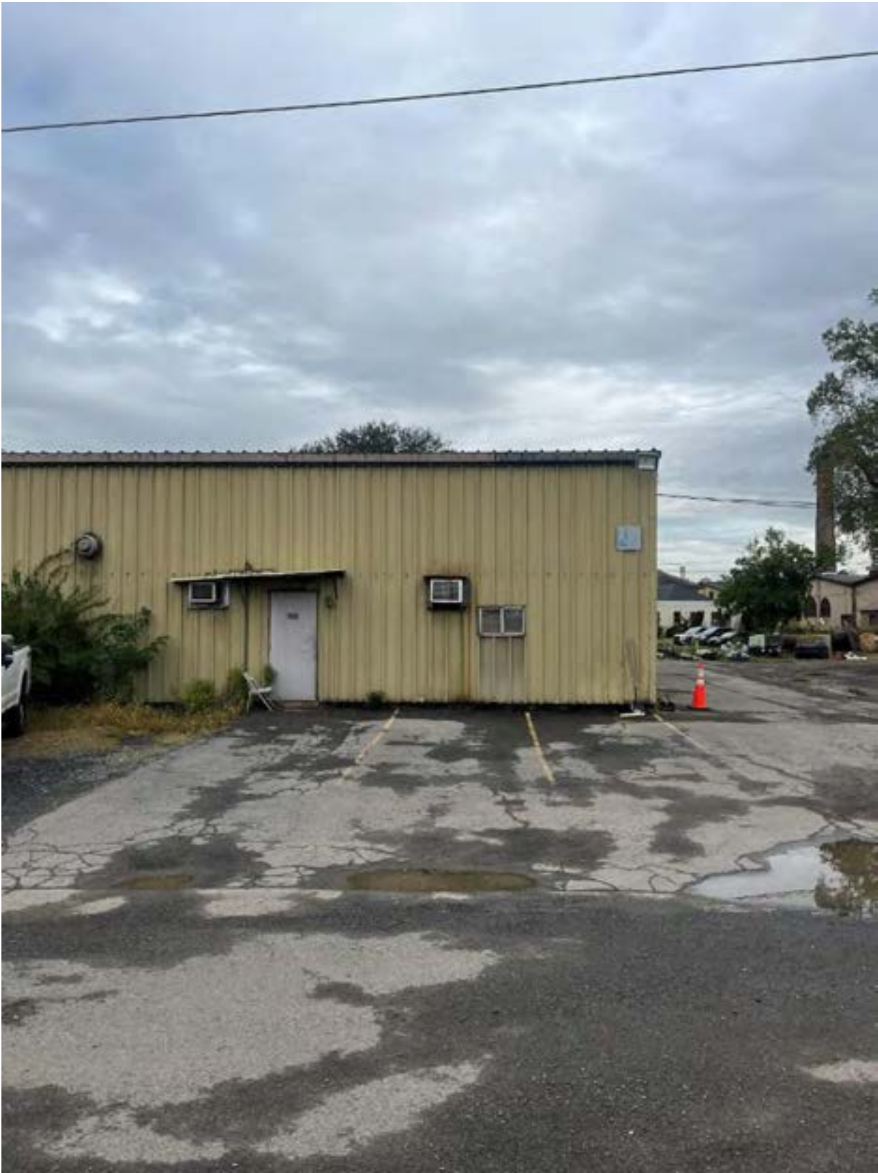
Pattern Shop – Building 24/27
