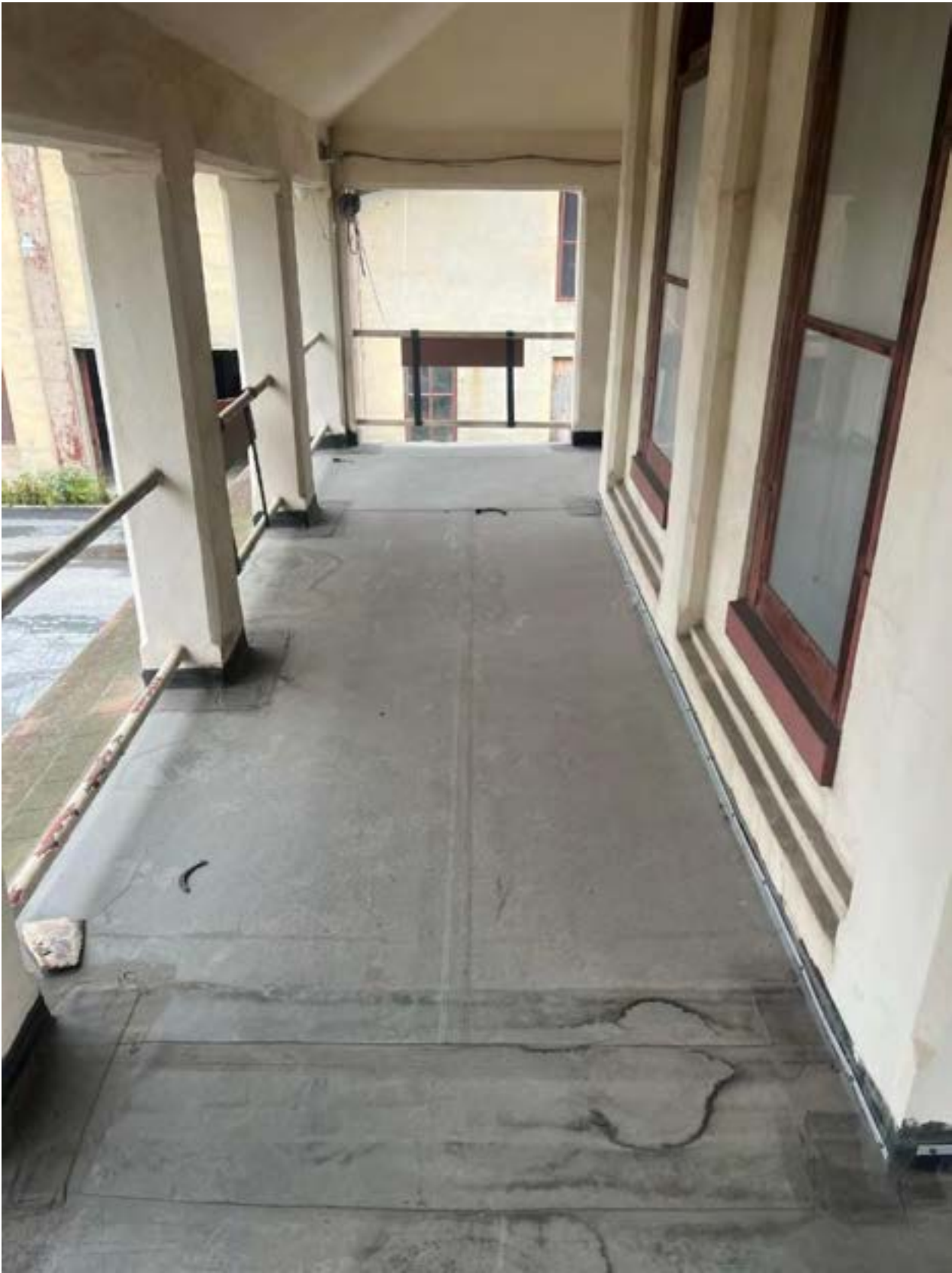
Building 3 - Window glazing.
