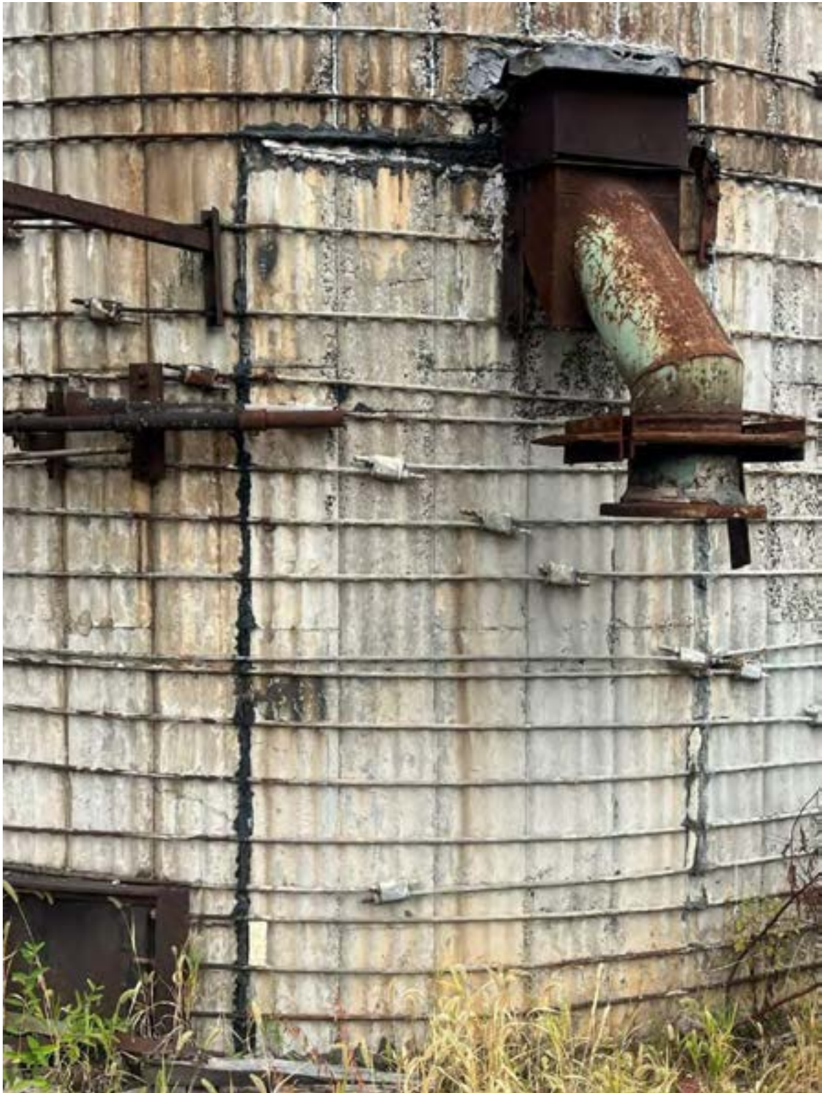
Silo - Tar Mastic
