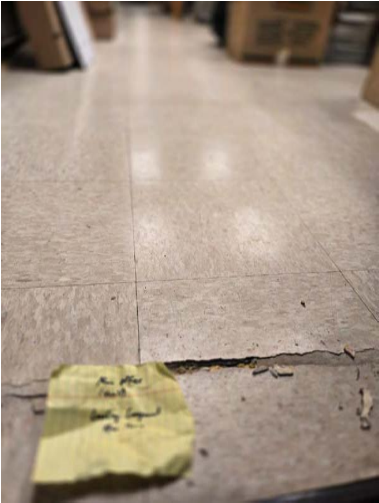
Building 3 – Leveling Compound
